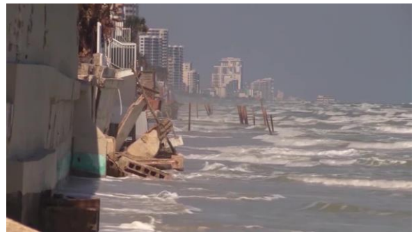
Picture 3: Rising sea levels destroy the foundation of our city! (Gonzalez, 2022)
